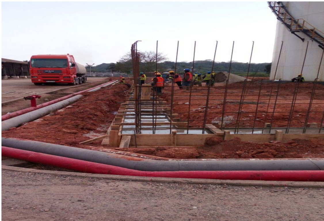
DIKE WALL CONSTRUCTION
