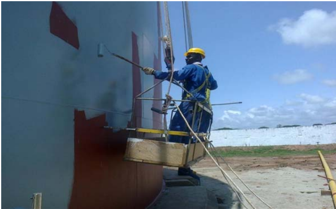
SAND BLASTING AND PAINTING WORKS
