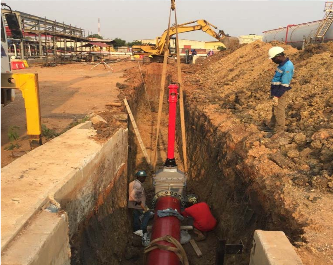
UNDERGROUND PIPING WORKS FOR RING MAIN
