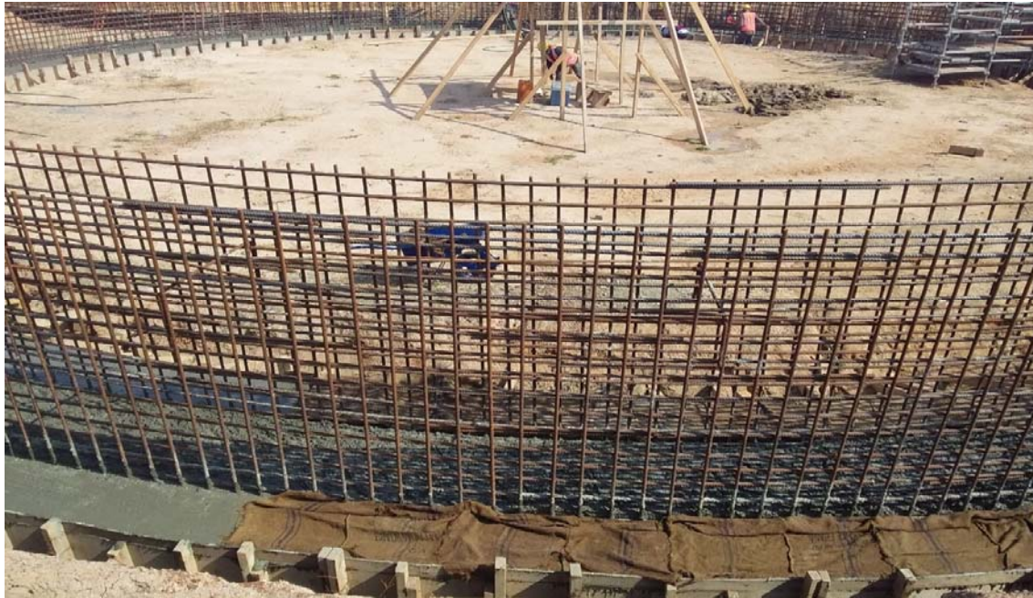
TANK FOUNDATION CONSTRUCTION WORKS
